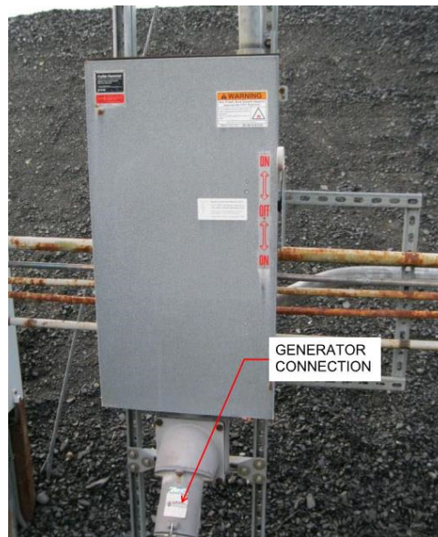
Generator Connection – (To Be Relocated and New Inlet Connection)
