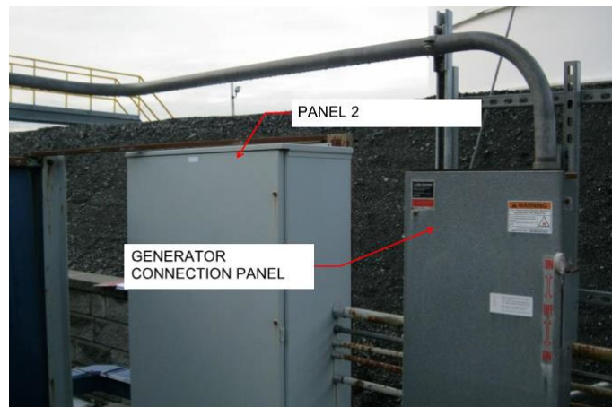
Generator Connection Panel
