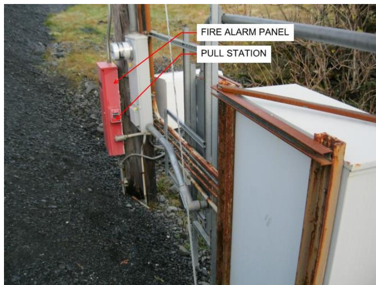
Panel 4: Fire Alarm with Pull Station
