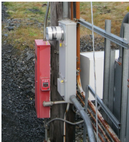
Existing 100A 208Y/120V Meter/Disconnect and Overhead Service Feeder
