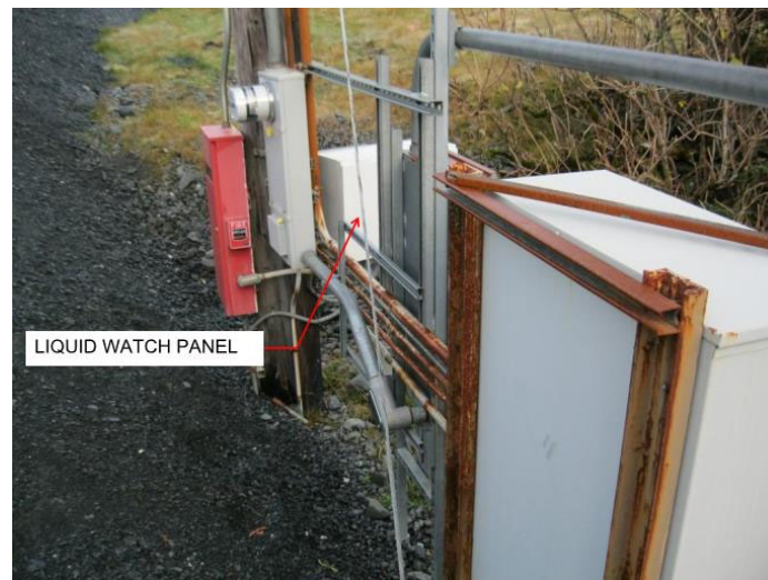
Panel 5: Liquid Sensor Panel
